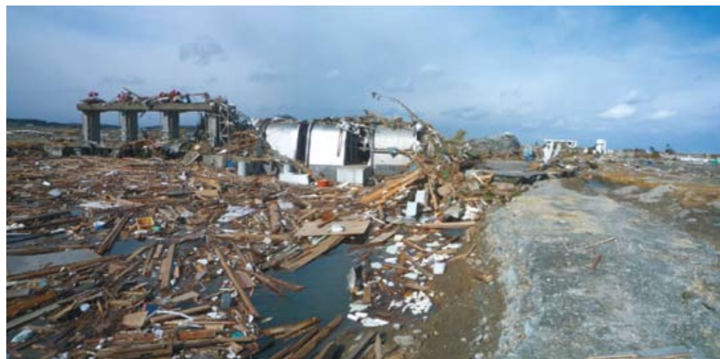
[大戸浜排水機場]
